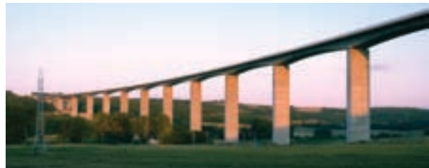
Kőröshegy viaduct and related section of M7 highway 68 400 tons of cement 180 000 m 3 of concrete
