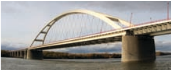
Pentele bridge 16 000 tons of cement 44 000 m 3 of concrete
