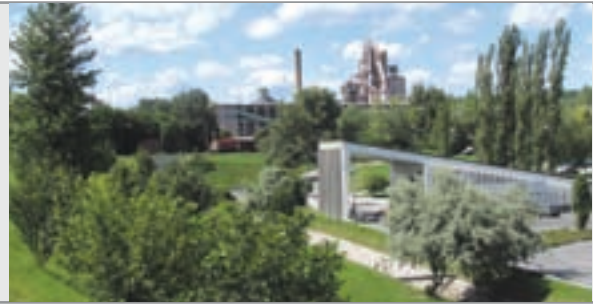
Vác plant from a bird's-eye view
