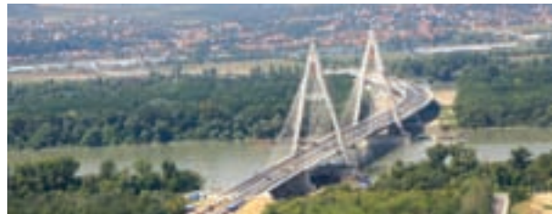
Megyer bridge 45 600 tons of cement 120 000 m 3 of concrete
