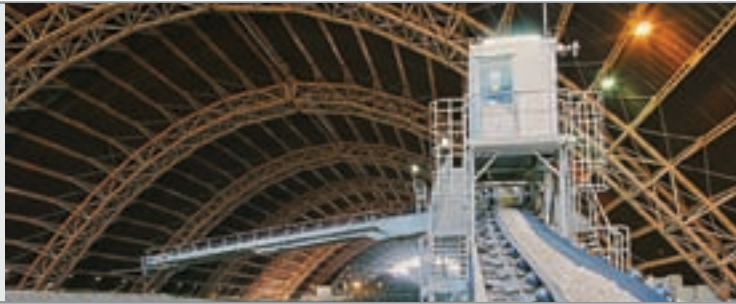
Mixing bed at the Vác plant
