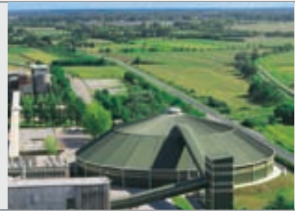
The Beremend plant
