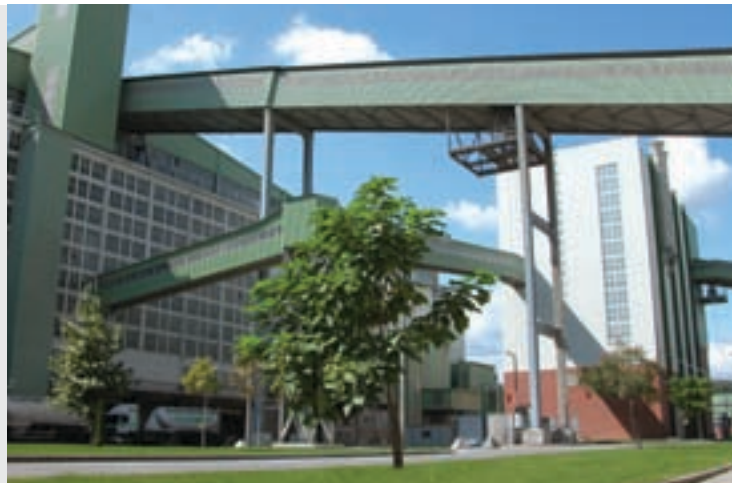
Packaging and grinding plant at the Vác plant
